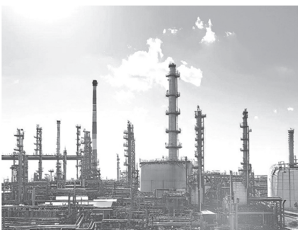
AI-generated refinery image
