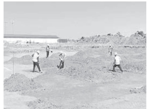
The construction site of the hospital at Number 75 Village
