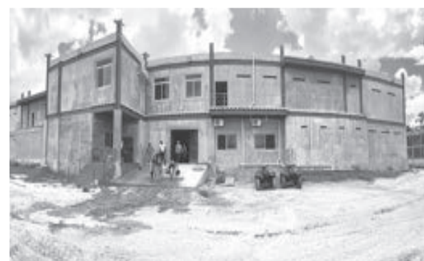
The construction of Mazaruni Prison Phase II has reached 75 percent
