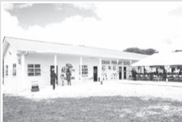
The Swan primary school, which was commissioned in November 2022
