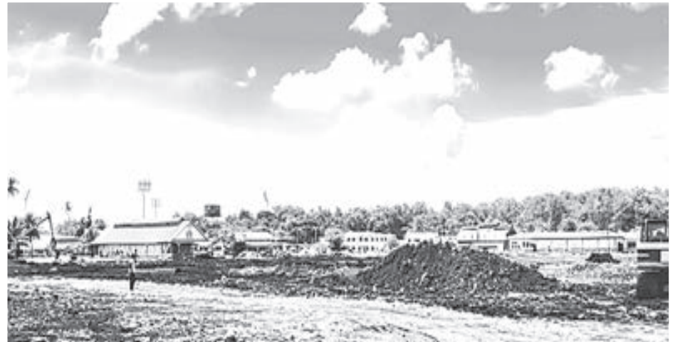
Land clearing commences for modern hospital at New Amsterdam
