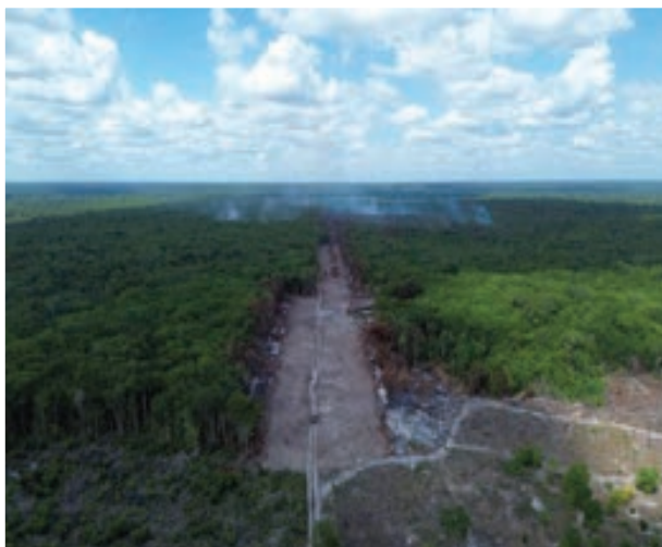
Land clearing has begun at Plantation York
