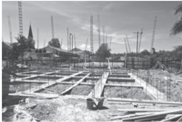
The ongoing reconstruction endeavours at the New Amsterdam Prison
