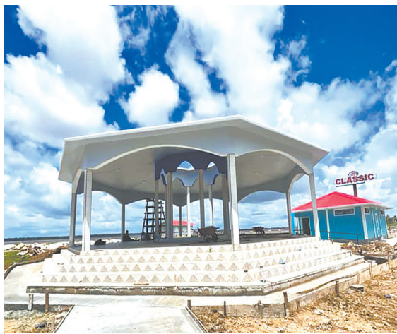
Bandstand being constructed at Corriverton recreational park
