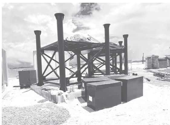
Works ongoing at the new Demerara River Bridge construction site
