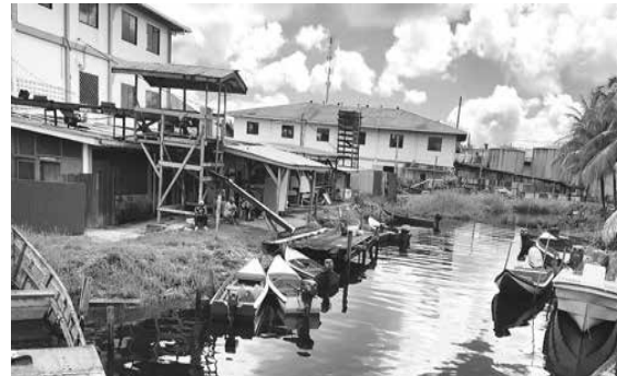
A $16.5M contract was signed for the construction of revetment at Charity
