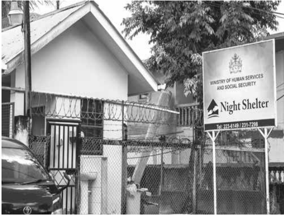
The shelter located at East La Penitence, Georgetown
