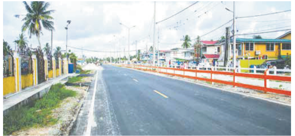
Part of the $1.4 billion Independence Boulevard (Punt Trench) enhancement project
