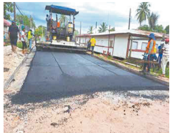
Ongoing infrastructural works in Central Kwakwani, Region Ten
