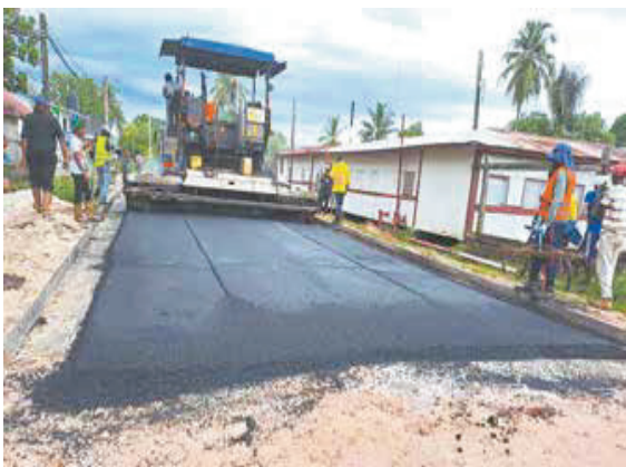
Ongoing infrastructural works in Central Kwakwani, Region Ten
