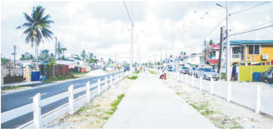
Part of the $1.4 billion Independence Boulevard (Punt Trench) enhancement project
