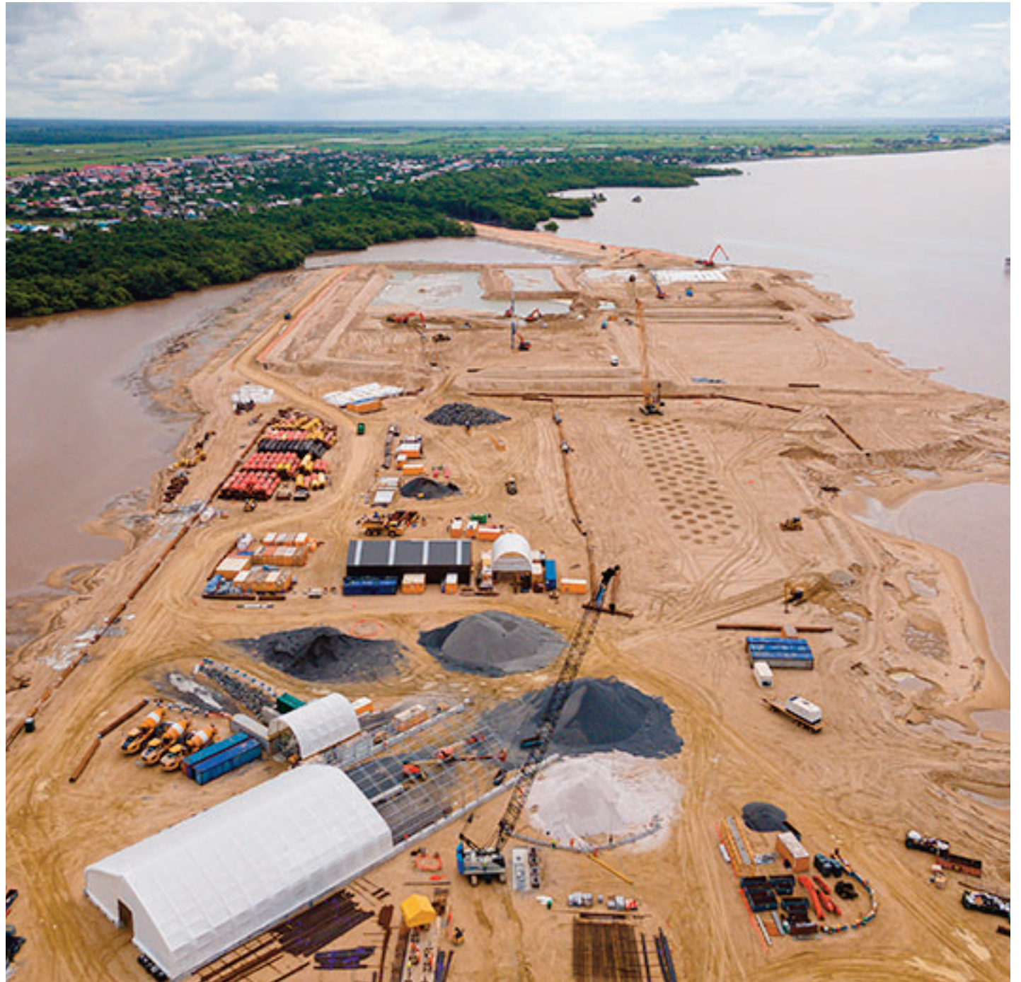
The artificial island being created by adding reclaimed material to the coastline
