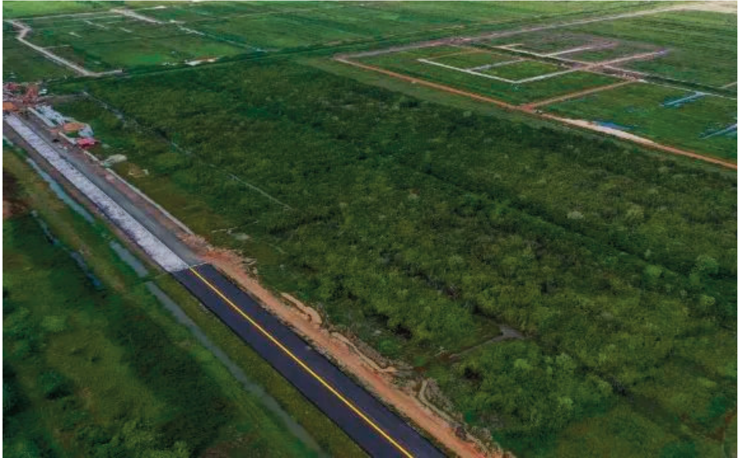
Aerial picture shows a highway being built into EBD
